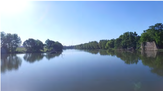
Figure 4a Emrichsville (16th Street) Dam in Indianapolis, IN. View from upstream, very difficult to see the low-head dam.
