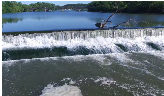
Figure 4b View from downstream. Discharge level was safe on that day.
