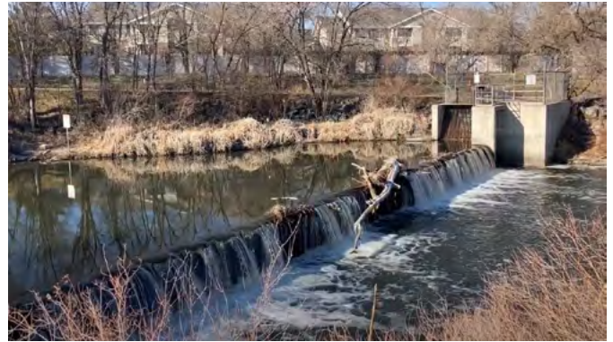
Figure 1 Low-head dam on the Jordan River in Taylorsville, Utah. A site with a single fatality. Note the warning sign on the left, well out of view of any recreationist, placed after the out-of-court settlement. The dam is now being replaced with recreational rock weirs.
