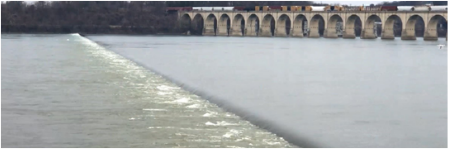
Figure 4. Photograph of Dock Street Dam
