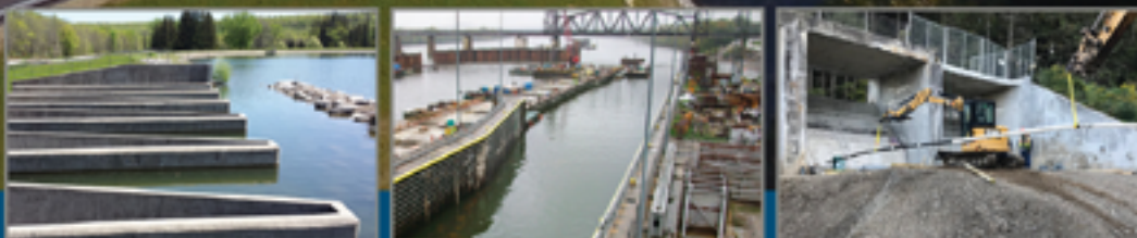
Red House Lake Dam
