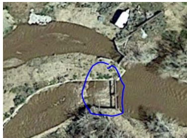
Figure 2: Example of a Low-Head Dam
