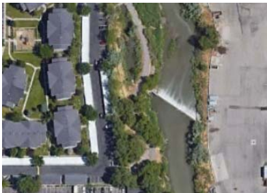
Figure 1: Example of a Low-Head Dam
