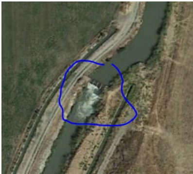
Figure 3: Example of a Low-Head Dam
