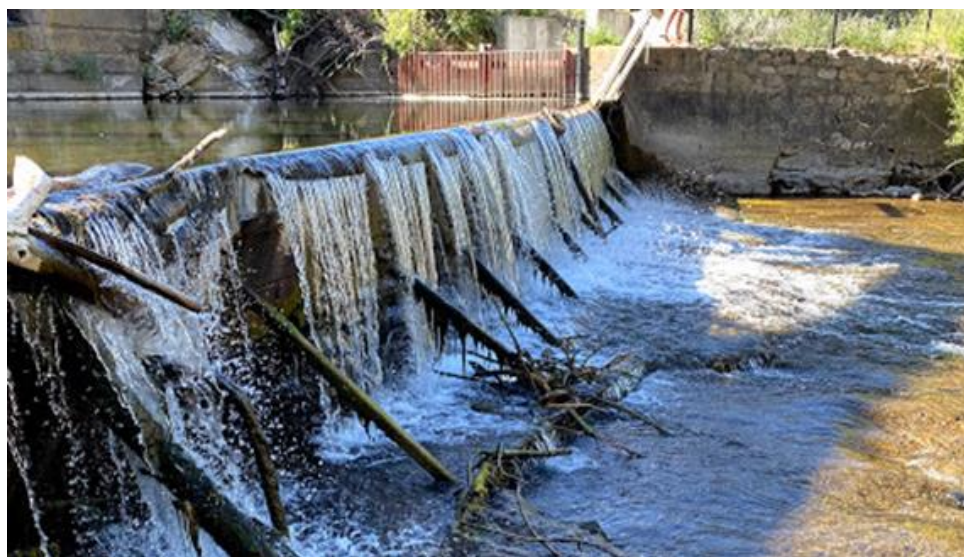
Figure 1. Low-head dam at Provo River by Provo Canyon (Photo by Salvador Vinay).
