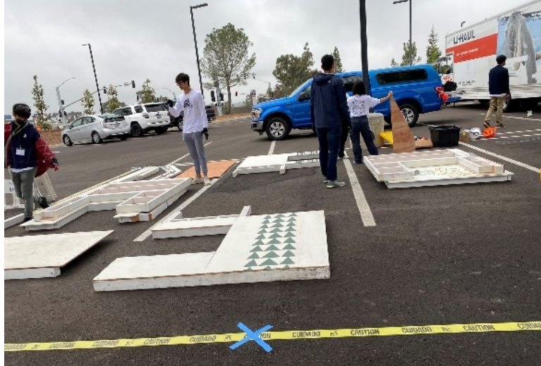
Example of panelized walls at 2022 TSDB
