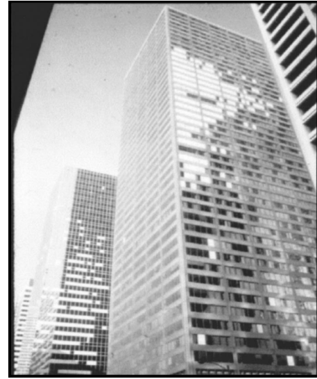
Fig. 3. Roof gravel blow-off caused window glass damage in Houston, Tex.
