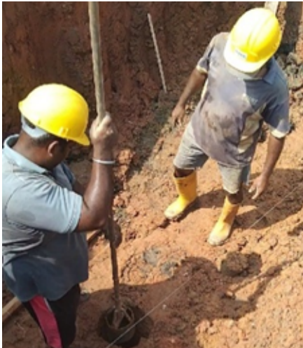
Figure 4 - make bore holes using shoring tool
