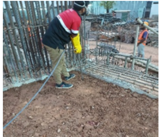
Figure 6 - insert termite chemical into soil
