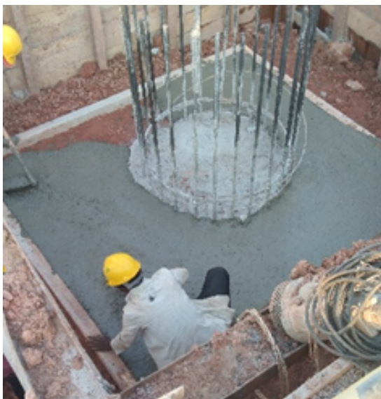
Figure 7 - pile cap screed concreting
