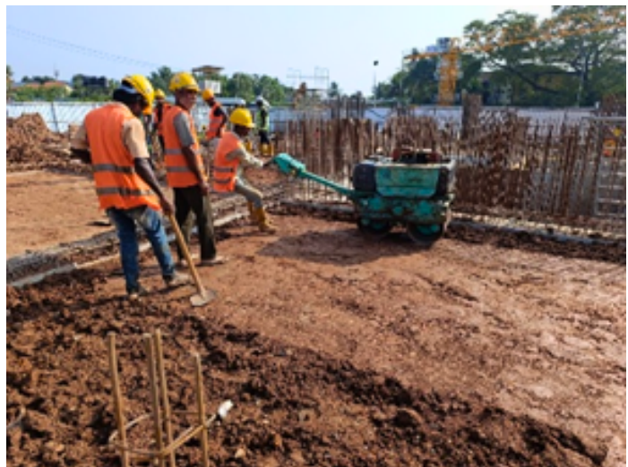
Figure 5 - compacting the soil using roller
