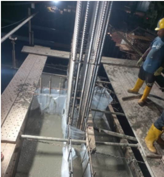
Figure 10 - pile cap concreting
