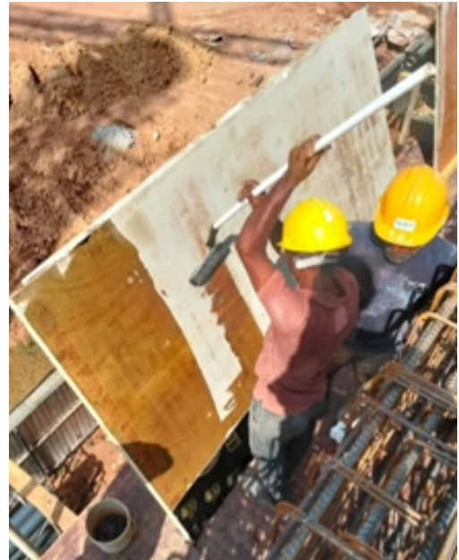
Figure 9 - applying demold agent to the side boards
