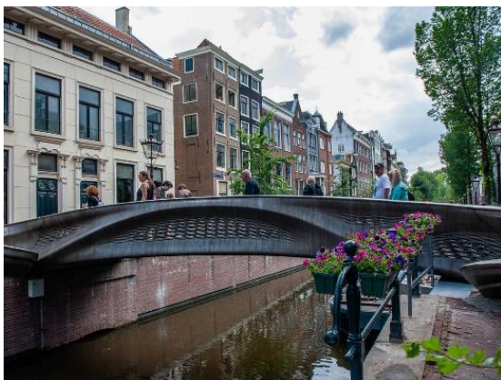
Figure 2: The world's first 3D printed footbridge , 2021, Amsterdam, the Netherlands (Ana Fernandez/SOPA Images/LightRocket via Getty)
