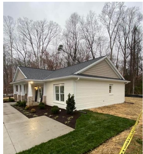
Figure: The first 3D-printed home in the United States , 2021, Williamsburg, VA (Alquist 3D)
