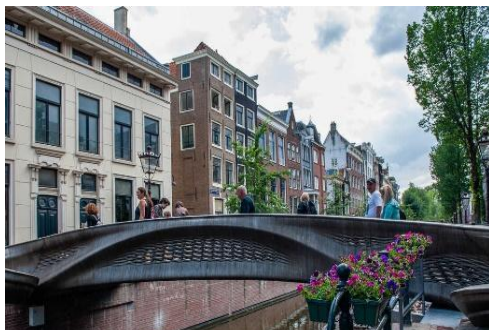
Figure: The world's first 3D printed steel footbridge , 2021, Amsterdam, The Netherlands (Ana Fernandez/SOPA Images/LightRocket via Getty)
