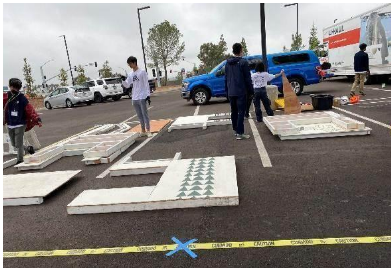
Figure 8: Example of Panelized Walls at 2022 TSDB
