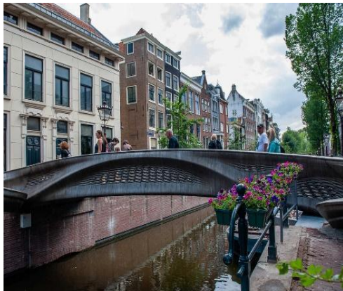
Figure: The world's first 3D printed steel footbridge, 2021, Amsterdam, The Netherlands (Ana Fernandez/SOPA Images/LightRocket via Getty)
