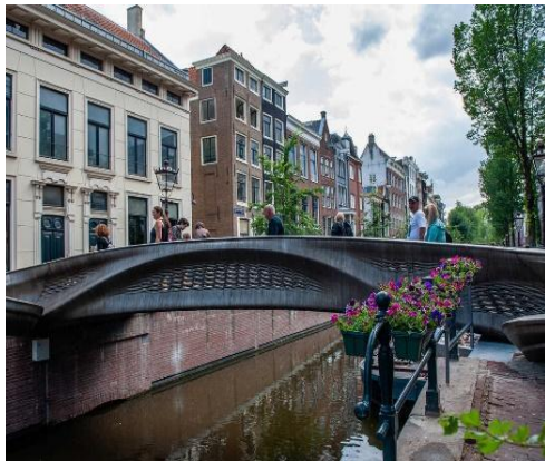
Figure : The world's first 3D printed footbridge , 2021, Amsterdam, the Netherlands (Ana Fernandez/SOPA Images/LightRocket via Getty)
