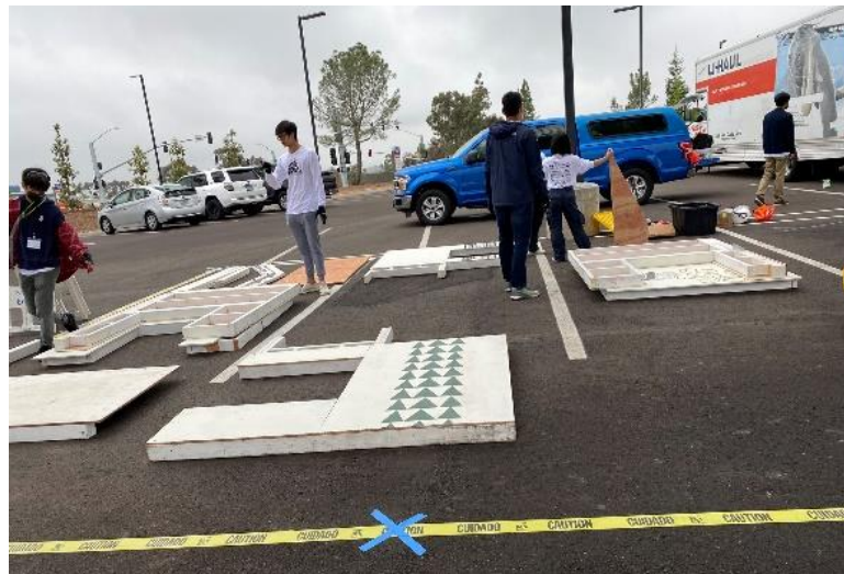
Example of panelized walls at 2022 TSDB
